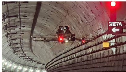
Tunnel inspection in Hongkong
